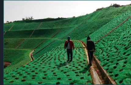
Project at CISUMDAWU TOLL ROAD, Jawa Barat
