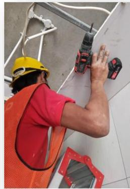
**Gambar 7.** Adjustment Panel Dinding dan Setting Kelistrikan
