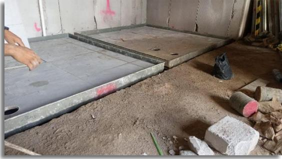
**Gambar 6.** Adjustment Panel Lantai
