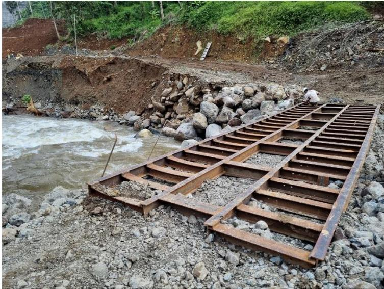
*Gambar 10 Setting Rangkaian H-Beam di Summer Bridge*
