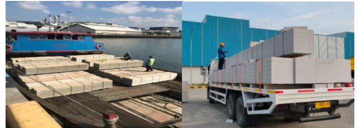
Gambar 4.1 Shipping/ Pengiriman Panel dinding AAC
