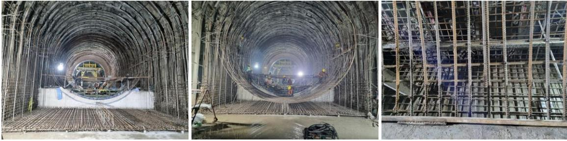
Gambar 4.5 Pembesian Lower Terowong Spillway Blok 21-50
