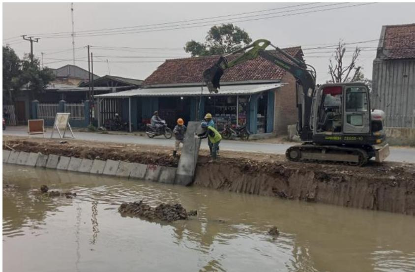
**Gambar 8 Pemasangan *Lining Tancap Pre-Cast***
