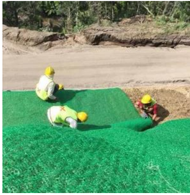
Gambar 1.1 Instalasi Material Geomat
