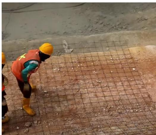
Gambar 1 Pemasangan wiremesh
